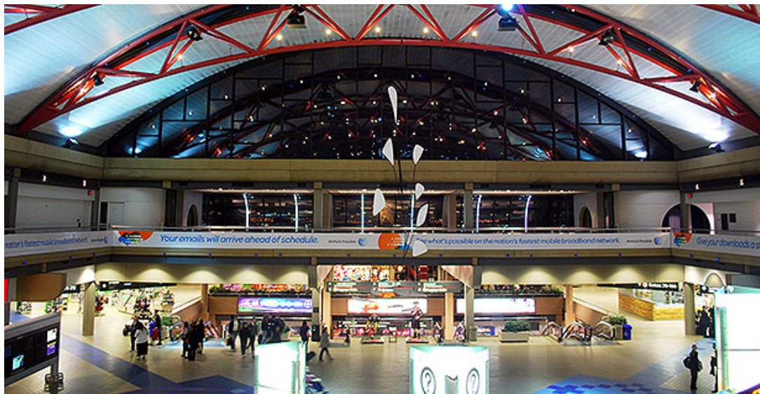
Pittsburgh International Airport is expected to be the first airport powered completely by a microgrid. John Marino/Wikipedia
